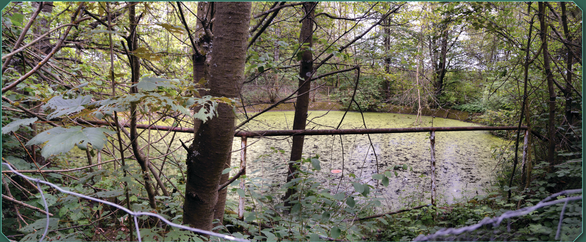
Charlie Battery Reservoir - 2018
